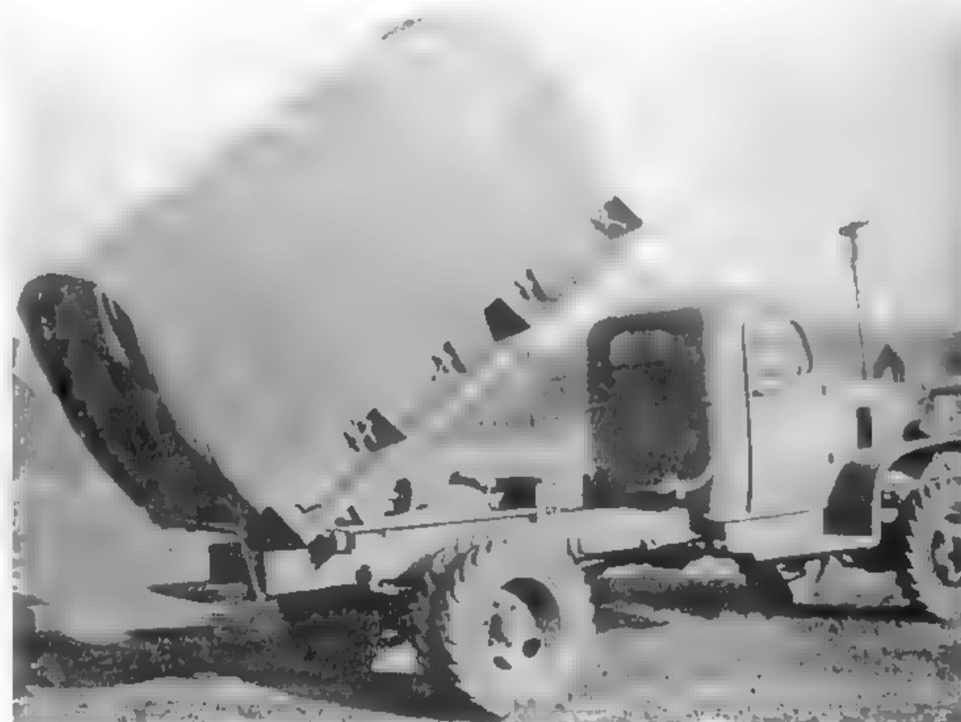
The G7106 dump truck was hard to distinguish from the standard cargo truck, until the bed was elevated as in this October 1941 Holabird Quartermaster Depot photo. (National Archives and Records Administration photo)
